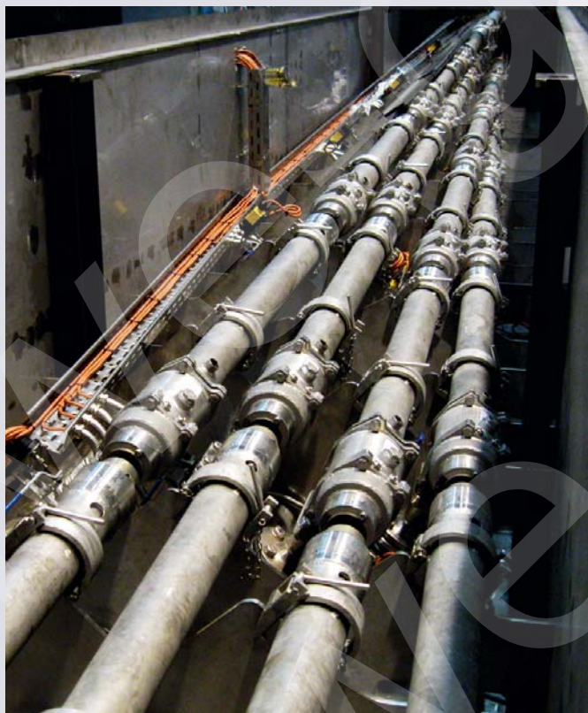
Four strand cooling pipe installation in special twisted mode.
